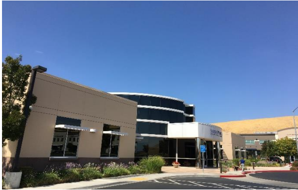
Light industrial new construction in unincorporated Contra Costa County
