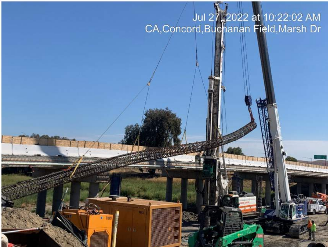
Figure 2 – Pile Cage Pick
