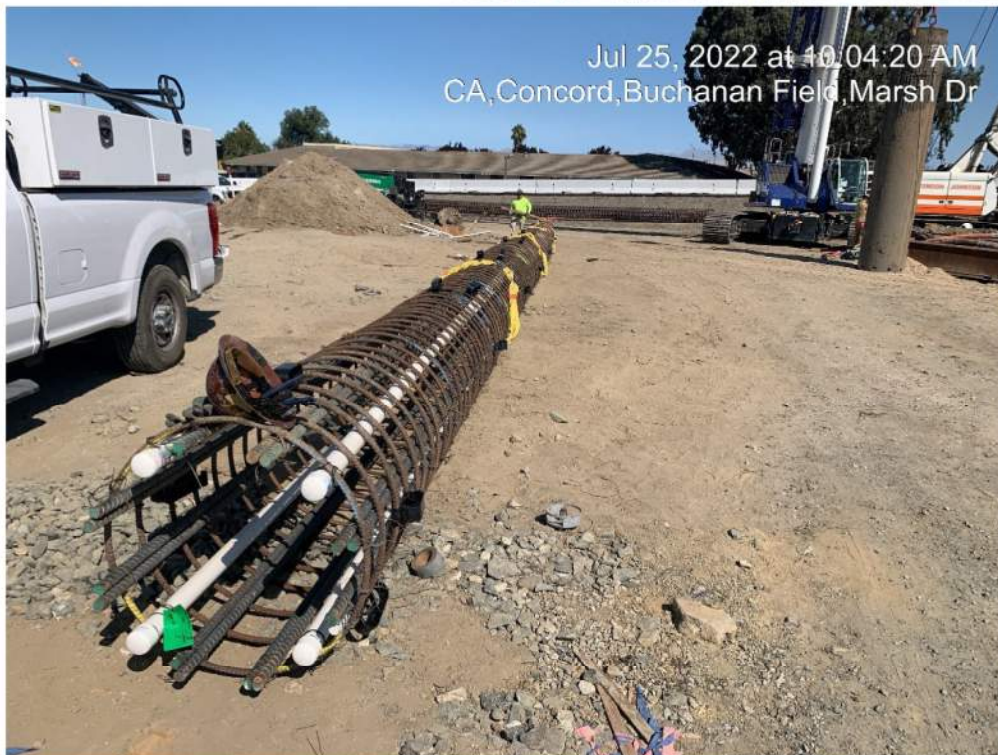
Figure 3 – Abutment 1 Piling
