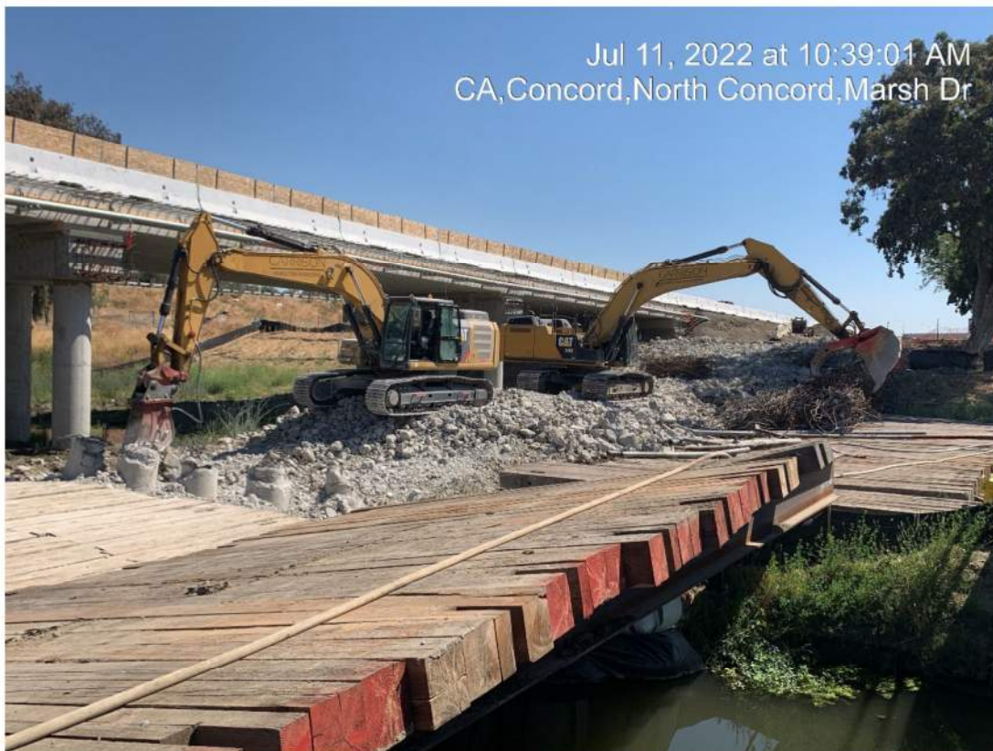
Figure 2 – Bridge Removal
