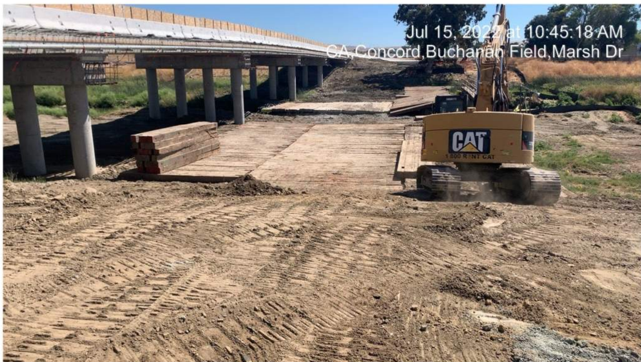
Figure 4 – Site Clean up
