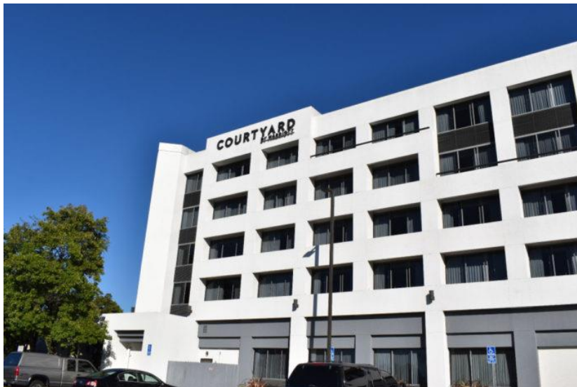
Courtyard Marriott at Hilltop is located at 3150 Garrity Way in Richmond.
